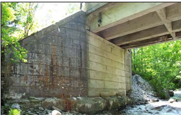
Bridge No. 8 Over Huntington River
