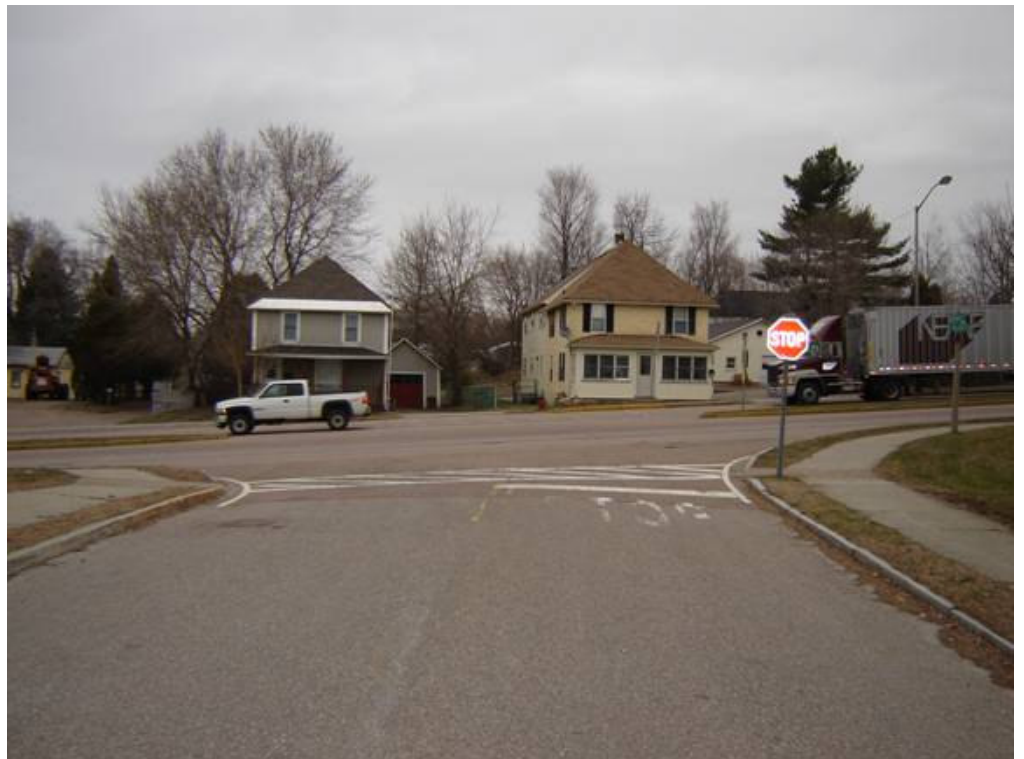
Figure 4. Roland Court, Looking North towards VT 15
