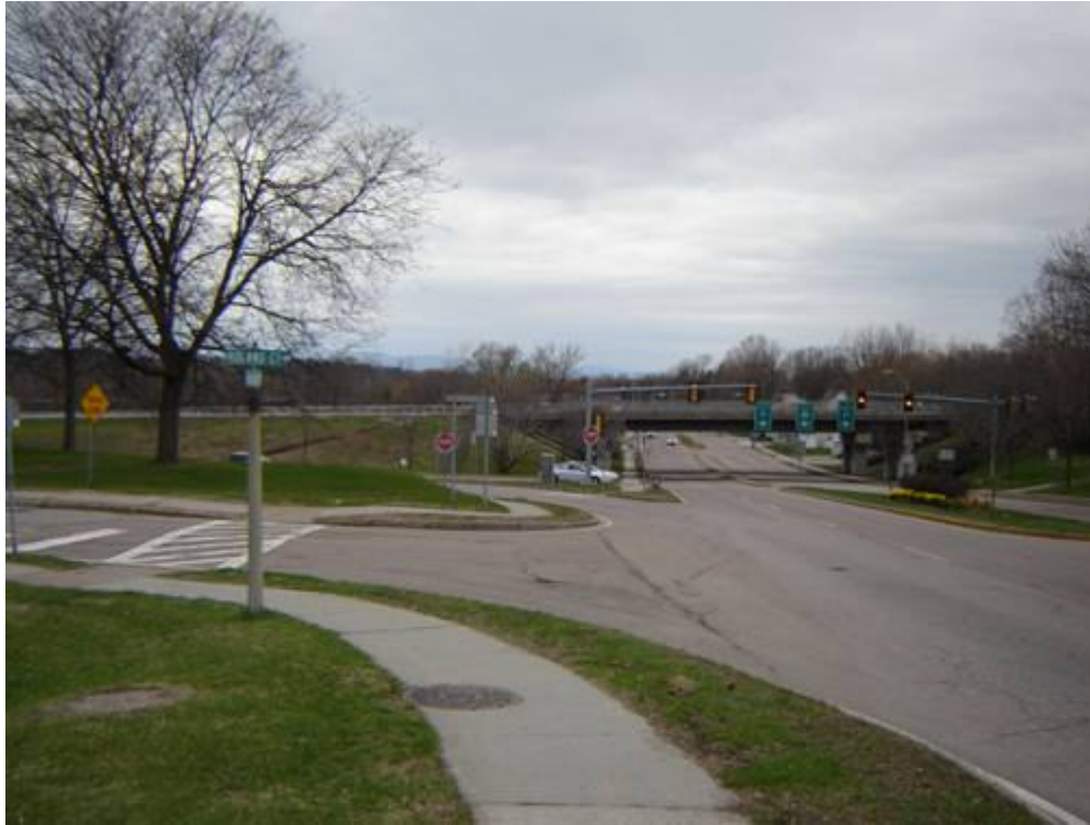
Figure 3. VT 15, Looking West (Roland Court is first on the left hand side followed by the I-89 slip lane)
