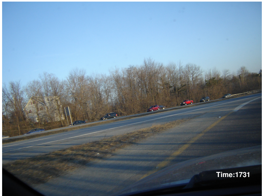
Figure 7. The Queue Extends Past the Gore Area into the Deceleration Lane on I-89 NB during the PM Peak (View is from the on ramp)
