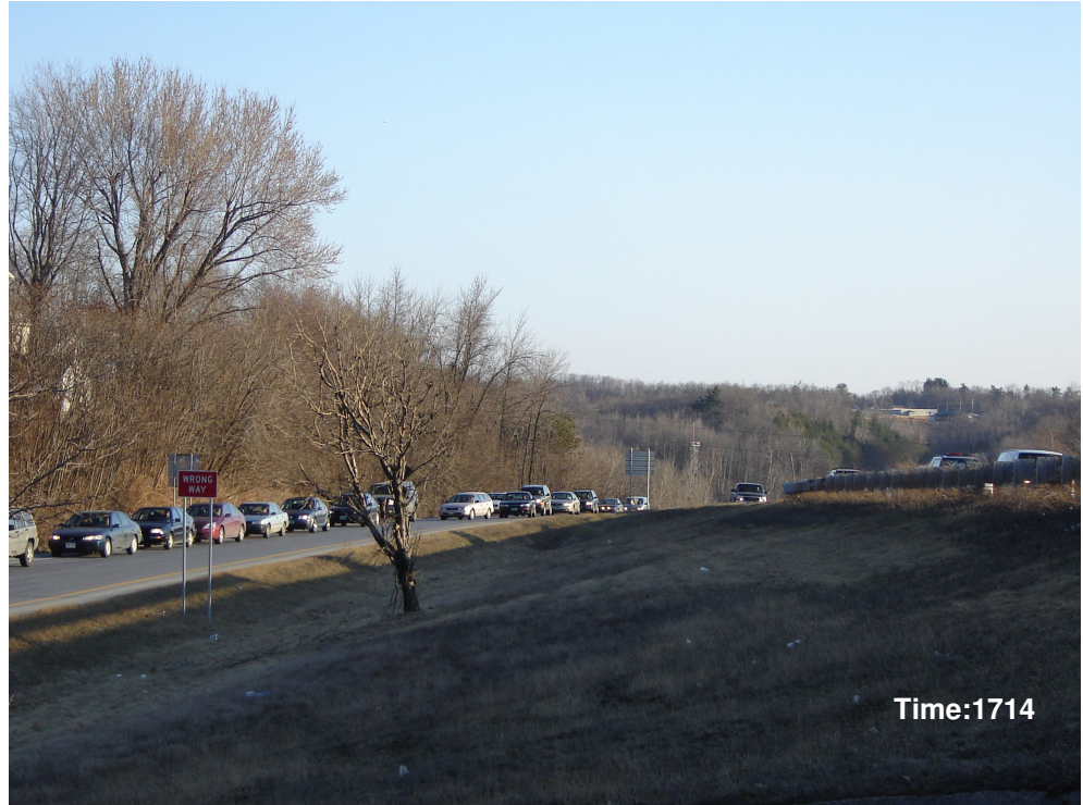
Figure 6. Right Turning Traffic Queues-up on the Off- Ramp during the PM Peak
