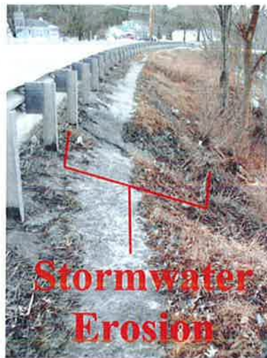
Figure 1.3. Site 2 Erosion of Footpath Due to Runoff
