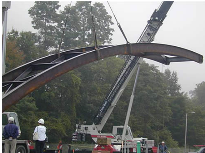
Waypoint Visitor's Center, Bellows Falls, Vermont
