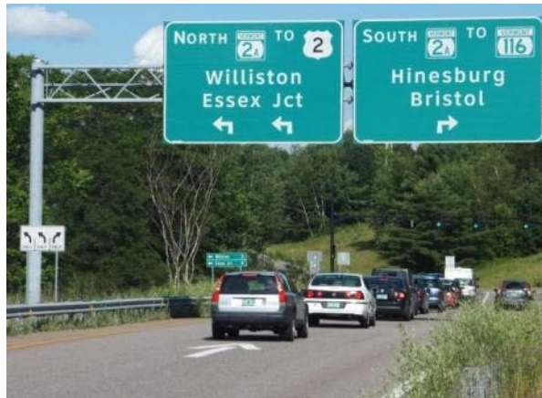
View of I-89 southbound off-ramp. Photo shows the relatively wide cross-section with limited pavement markings to designate lane use. A queue is building in the center lane that serves as a shared thru-left, while the left-most lane is under-utilized.
