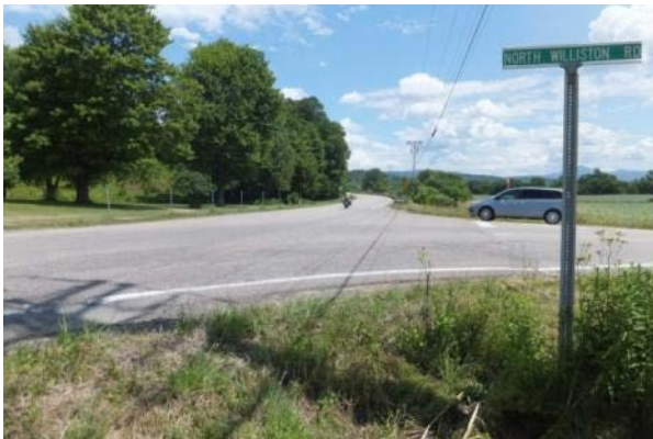
View of the intersection looking east. Photo shows the limited sight distance to the east due to the horizontal curve and vegetation.
