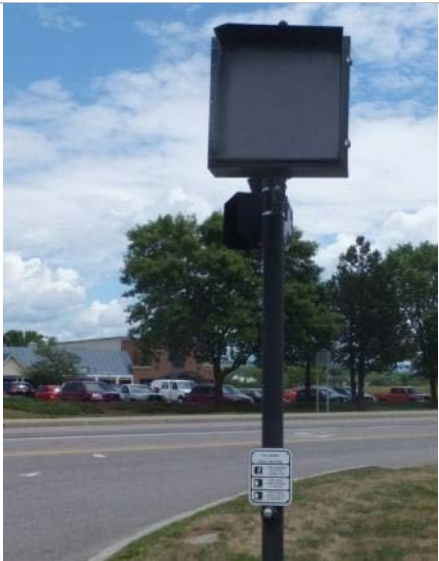
Photo shows the no right-turn-on-red sign “blacked-out” when the pedestrian phase is not activated.
