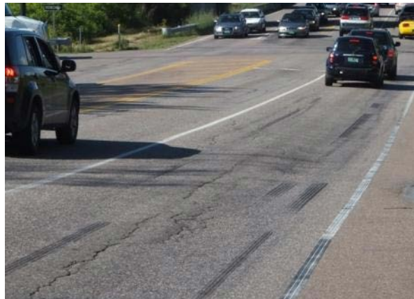
View of I-89 southbound off-ramp. Photo shows the relatively wide cross-section with limited pavement markings to designate lane use. A queue is building in the center lane that serves as a shared thru-left, while the left-most lane is under-utilized.
