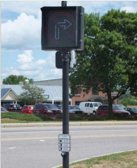
Photo shows the no right-turn-on-red sign activated when the pedestrian phase is activated.
