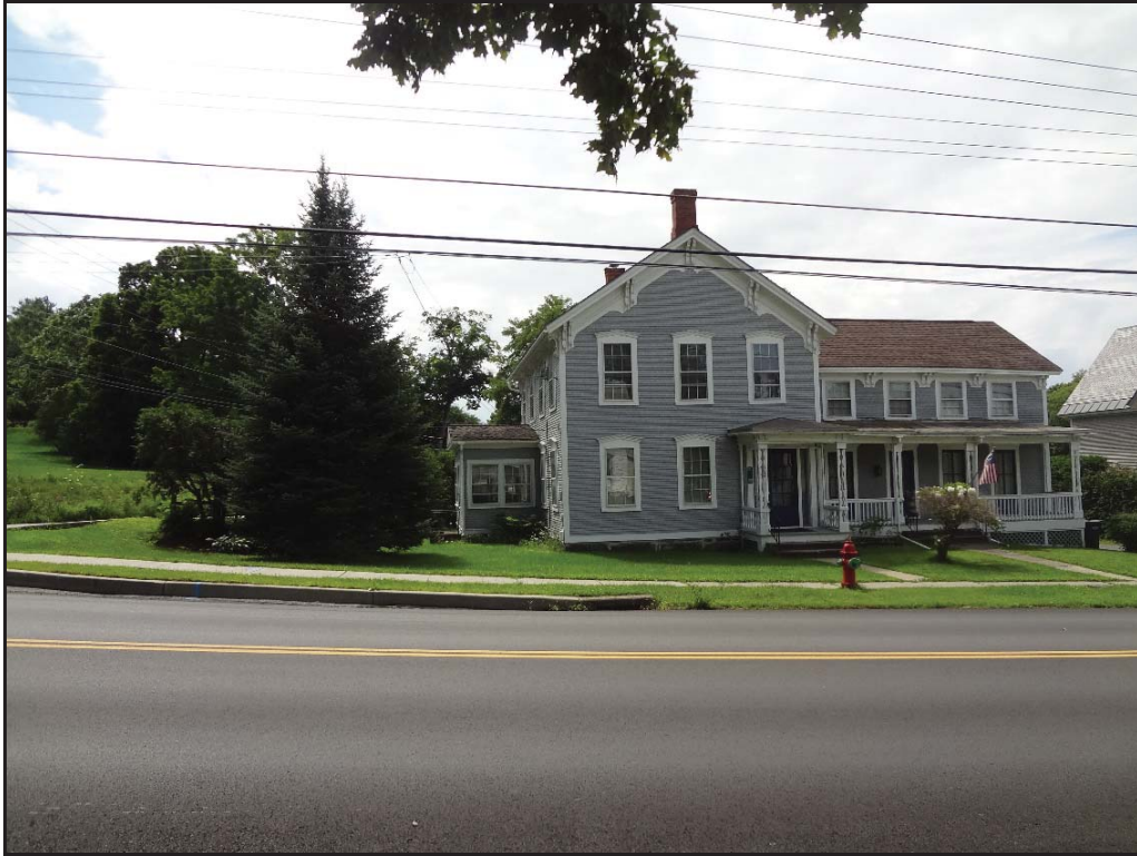
Photo 9. Structure 1, 79 Main Street, facing south. A wood-framed T-plan house of 1 1/2 stories with Italianate details.
