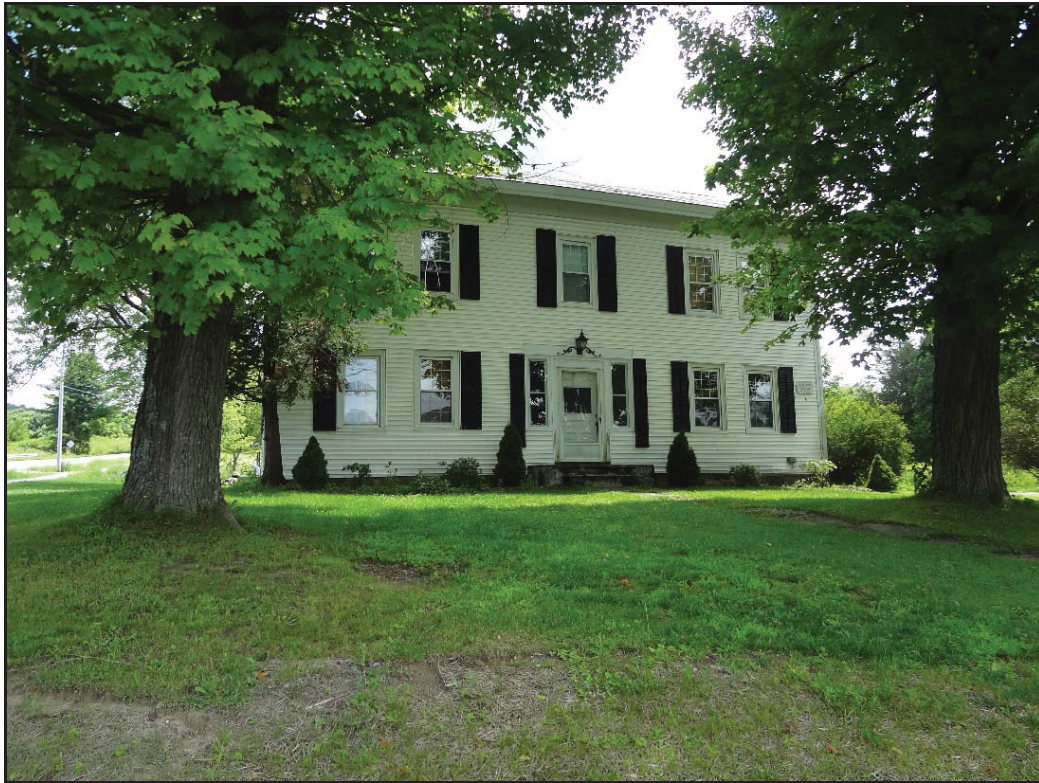
Photo 16. Structure 8, 4 East Road, facing northwest. A 2-story 5-bay wide center-passage vernacular wood-framed house with gable roof.
