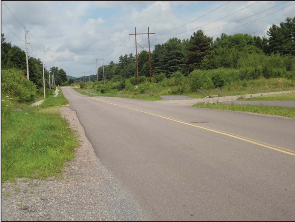
Photo 1. Photo shows a view of Area 1 - Haydenberry Drive north of McDonalds. View is to the north.
