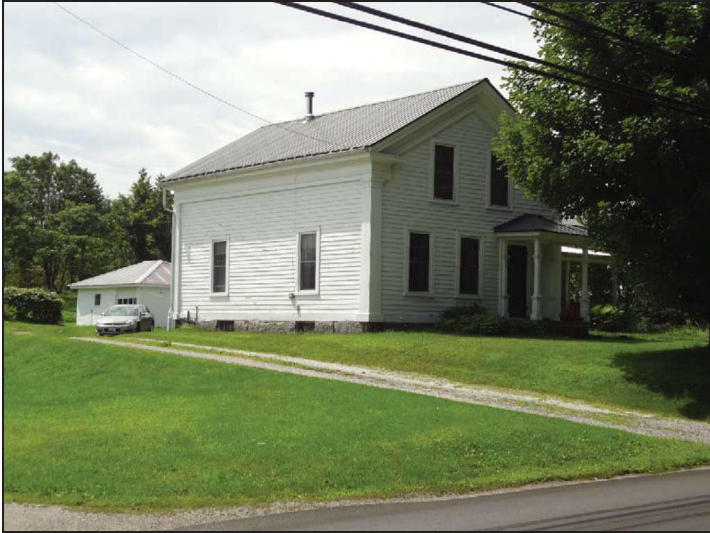
Photo 11. Structure 3, 89 Main Street, facing southwest. A 1 1/2 story wood-framed Greek revival upright-and-wing house with associated outbuildings.
