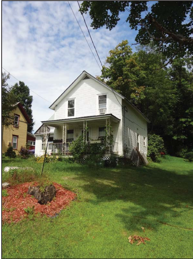
Photo 14. Structure 6, 96 Main Street, facing northwest. A 2-story wood-framed gable-entry vernacular house with 1 1/2 story addition forming a T plan.
