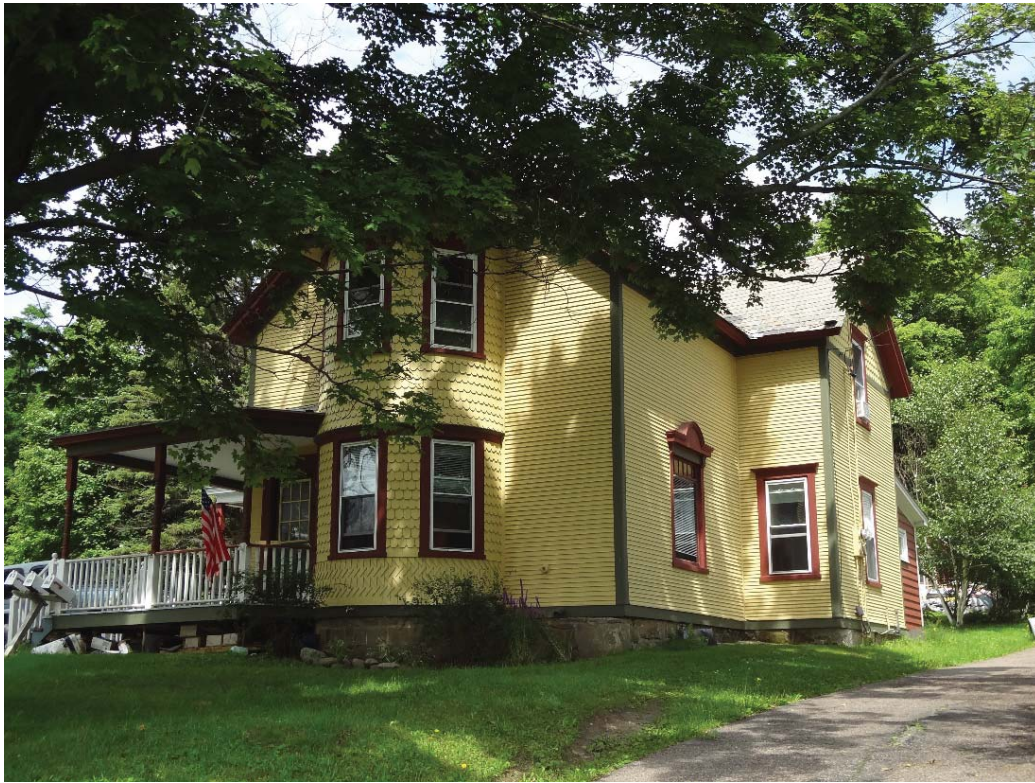
Photo 13. Structure 5, 94 Main Street, facing northwest. A 2-story wood-framed Queen Anne style house with intersecting gable roof.
