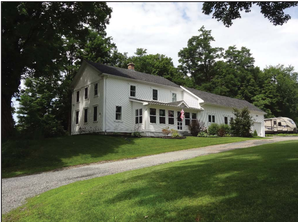
Photo 12. Structure 4, 88 Main Street, facing northwest. A 2 story wood-framed vernacular house with gable roof and 2-story garage addition.
