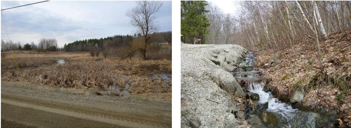
**Figure 2.** Left: A high-scoring segment, low slope segment of Lost Nation Road in Essex. Right: A high-scoring, high slope segment of Lower English Settlement Road in Underhill, where a stream channel flows alongside the road with greater risk to water quality.
