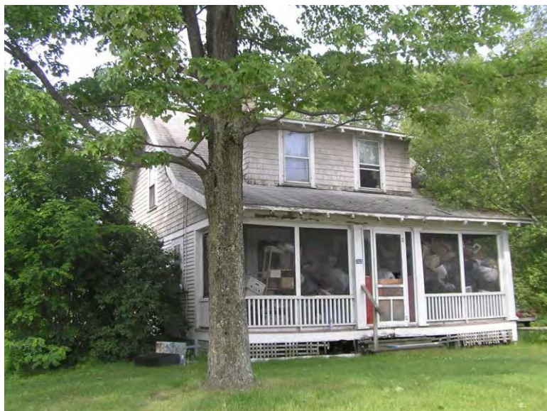
4. Front elevation of 202 Colchester Road with rafter tails, battered porch posts, front yard and trees.
