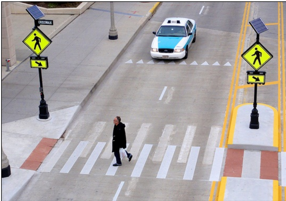
Figure 11: Example of Crosswalk Highlighted with Rapid Flashing Beacons and Signage
