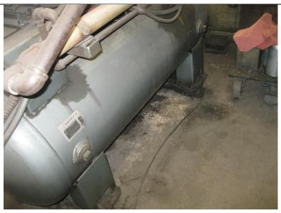
Photograph 9: Compressor room in 50 Lakeside Avenue building. Note oil staining on floor.
