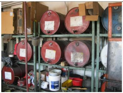
Photograph 3: Hydraulic oil and lubricant storage in former paint room. Heavy staining was evident on floor.
