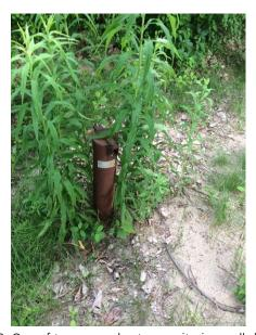
Photograph 20: One of two groundwater monitoring wells located in northernmost portion of Subject Property.
