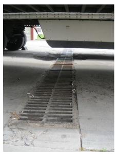
Photograph 10: Storm drain in loading dock area of 50 Lakeside Avenue building.
