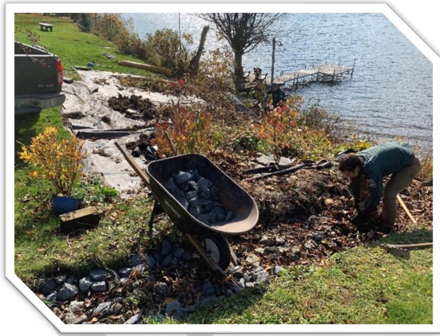
Figure 18. Vermont Youth Conservation Corps installing a no-mow buffer and stone-lined channel to infiltrate and slow runoff from impervious surfaces on the Lake Elmore shoreline (Photo by Peter Danforth).
